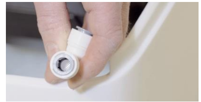
Replacement of brine discharge elbows
